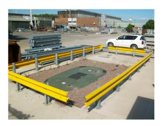
**Crash Barriers** can be used to protect your stock, plant and buildings from damage caused by fork lift trucks and slow moving vehicles.
